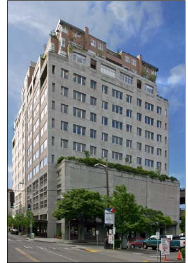
Waterfront Place Building Seattle, Washington
